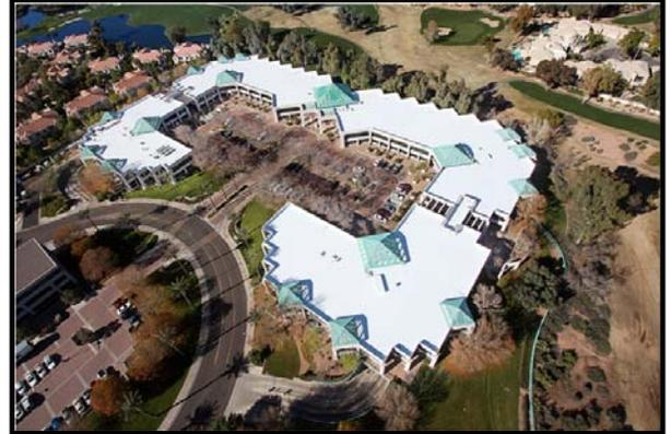
The original roof system was a [ballasted EPDM](#) blanketed by 2" of river rock. The new system installed by [Starkweather Roofing](#) in December 2008 was finished with a white [PolyKool cap sheet](#). And is capable of withstanding Arizona's extreme
